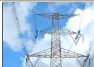
Switching & Lightning Protection Using Externally Gapped Line Arresters
