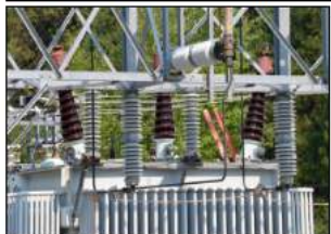
Using Dielectric Frequency Response to Assess Bushing & Instrument...
