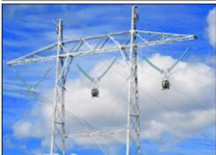
Glass Insulators Used for Network Expansion at Norwegian TSO
